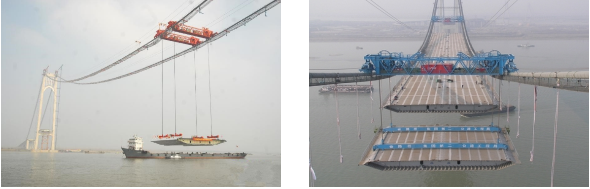
FIGURE 9. Placement of the deck segments during the construction of suspension bridge.
