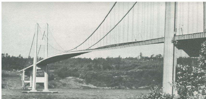
Figure 2: Wide oscillations at the collapsed Tacoma Narrows Bridge (1940).
