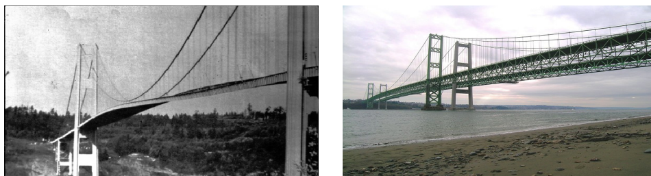
FIGURE 5. The collapsed Tacoma Bridge and the current twins Tacoma Bridges
